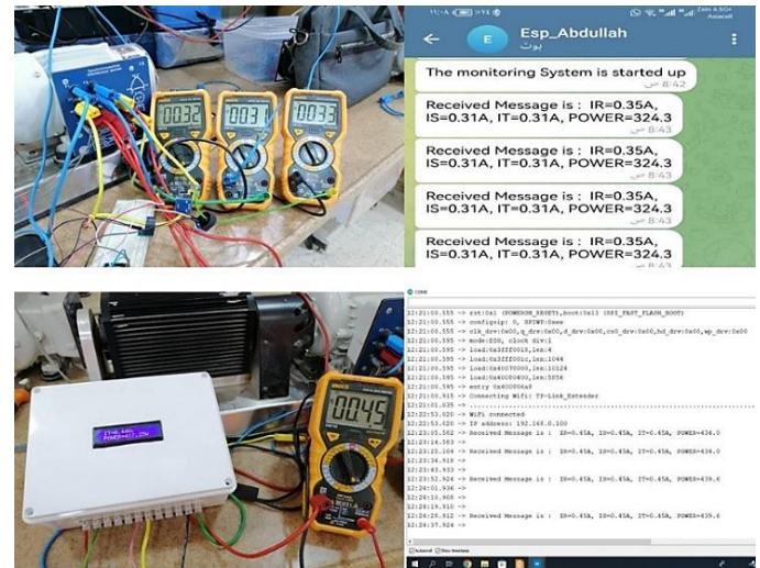
Figure 7: Monitoring system with load
