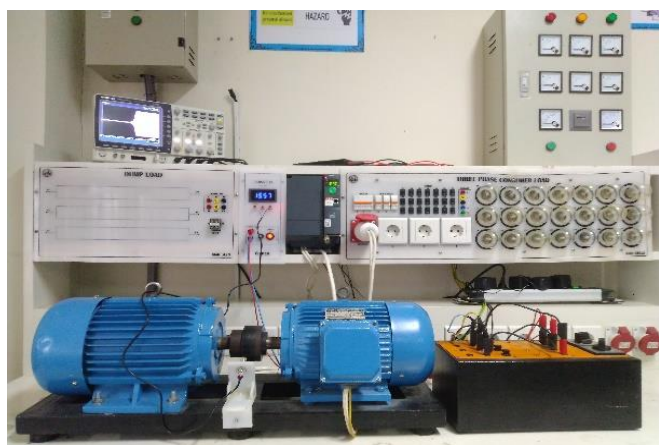
Figure 5. Experiment setup for SEIG for various operating conditions
