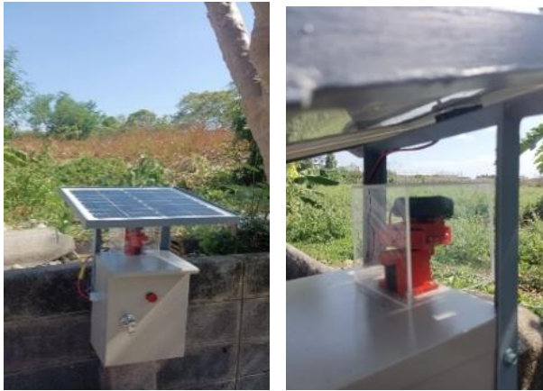
(a) Installation of system position 1 and 2
